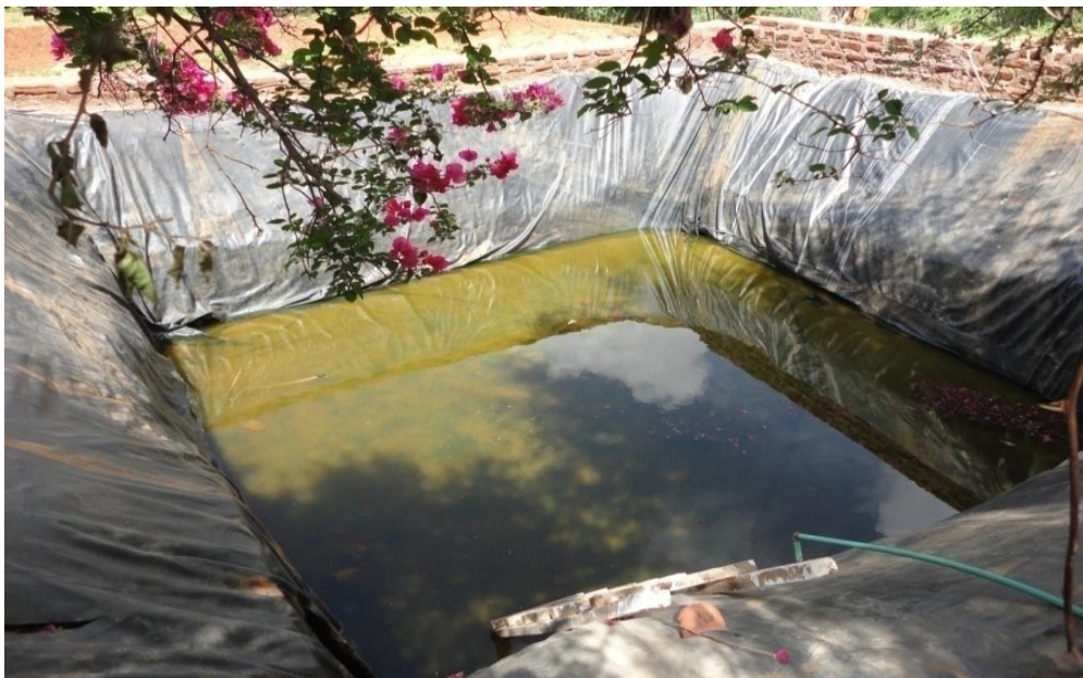
Plate 4: Fishpond under construction near Mwingi Town of Kitui County, Kenya
